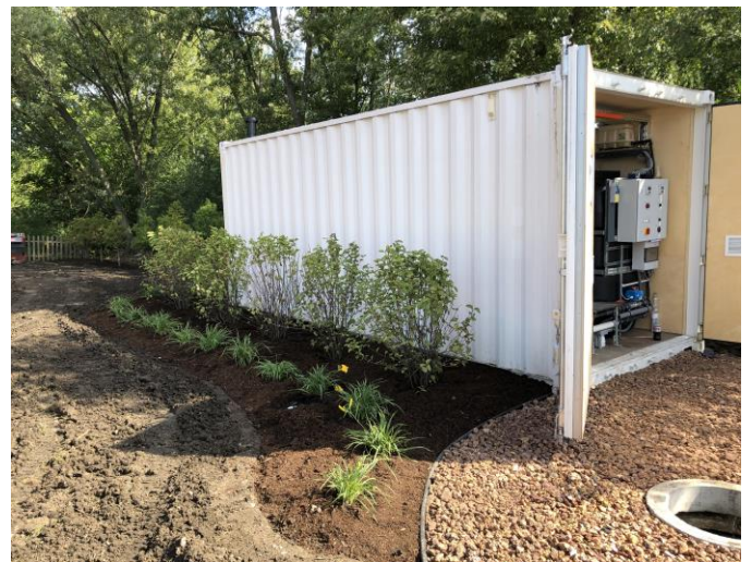
Exterior view of the container plant
