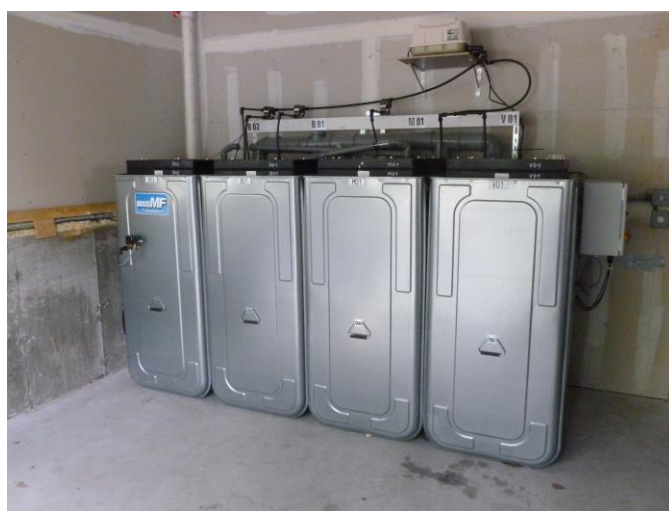
Assembly of the BUSSE-system Type GT 440.
