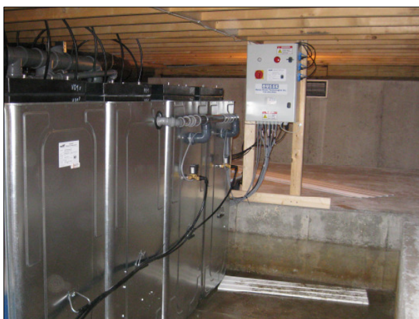
Installation of the system in the basement
