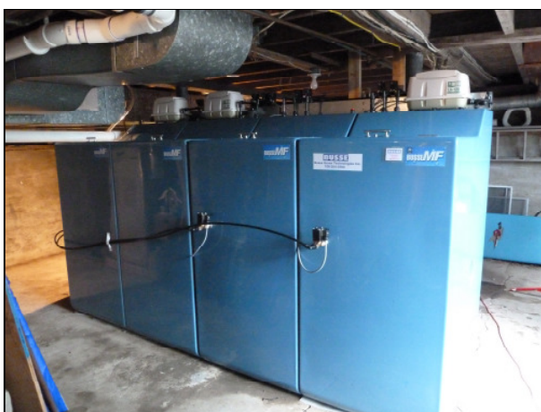
Installation of the system in the basement
