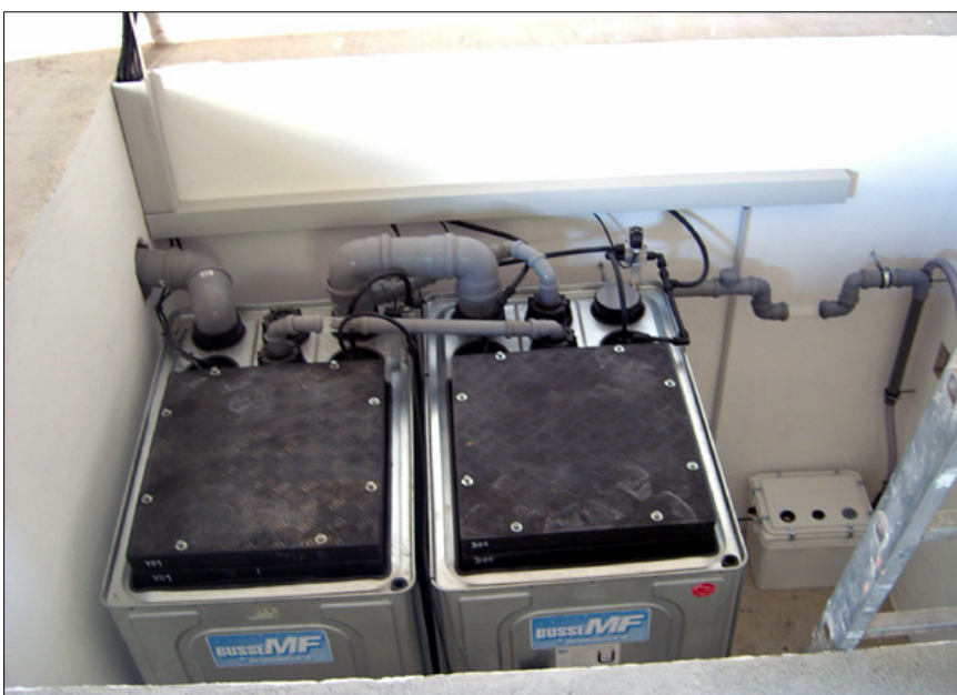
Waste water treatment system
