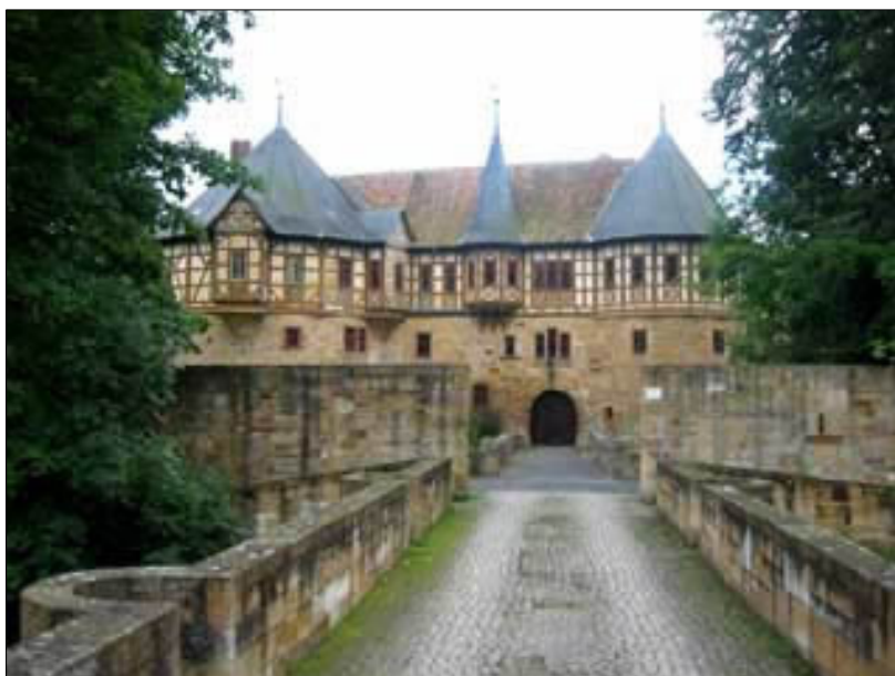
View of castle Irmelshausen
