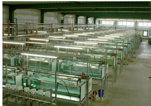
Pilot project „effluent free aquaculture“ in Thierbach - line of 6 breeding systems
