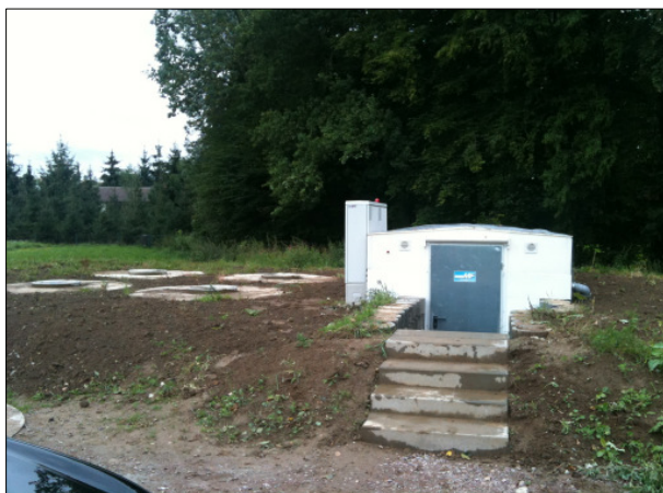
Underground module with septic tanks
